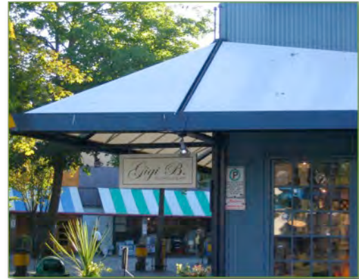
Awnings provide weather protection for sidewalks.
